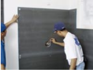
Cuts out are easily made using a utility knife or a jigsaw.
