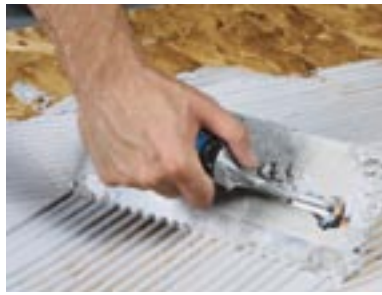
Simply spread polymer modified mortar over a clean wood subfloor.
