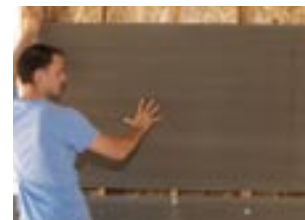
Positioning lightweight wedi building panel is
