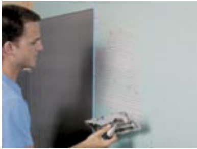
Trowel a bed of modified mortar over the wall.
