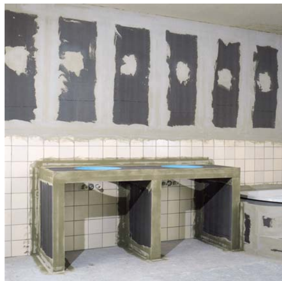
Pictures 3 – 4 One or two layers of 2" wedi Building Panel are installed as the horizontal sink carrying board. They are adhered to the vertical panels using wedi Joint Sealant and wedisteck Connectors to achieve quicker stability of the assembly.
