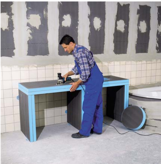
Pictures 3 – 4 One or two layers of 2" wedi Building Panel are installed as the horizontal sink carrying board. They are adhered to the vertical panels using wedi Joint Sealant and wedisteck Connectors to achieve quicker stability of the assembly.
