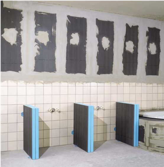
Pictures 1 – 2 2" wedi Building Panels are used for vertical support of the washstand. The panels are adhered using modified thinset mortar and mounted against the wall using wedisteck connectors.
