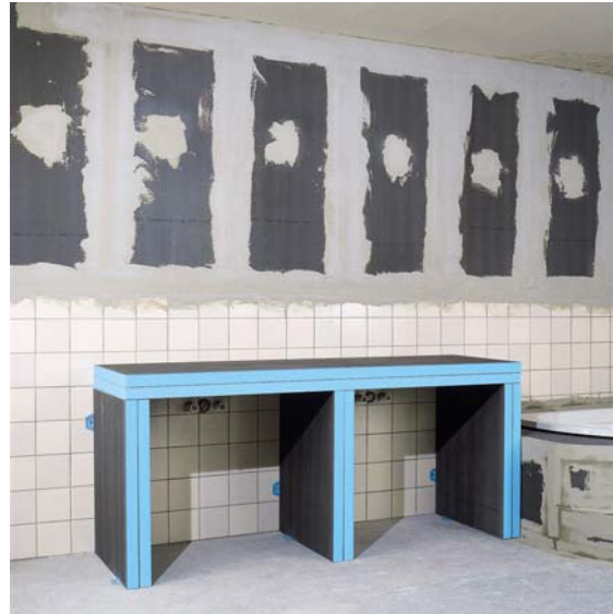
Pictures 1 – 2 2" wedi Building Panels are used for vertical support of the washstand. The panels are adhered using modified thinset mortar and mounted against the wall using wedisteck connectors.
