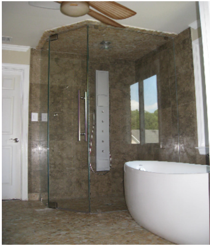
Picture 3: The barrier free shower is tiled and ready for use
