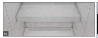
After 24 hours, tiling can commence to include the underside of the bench.
