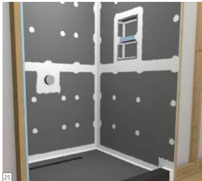
**EN** Weight is applied for a minimum of 30 minutes on and against the curb (from outside) and another 1/2 in. bead of sealant is applied over all curb seams and spread flat. The seams must be covered 1 in. either side of a seam.
