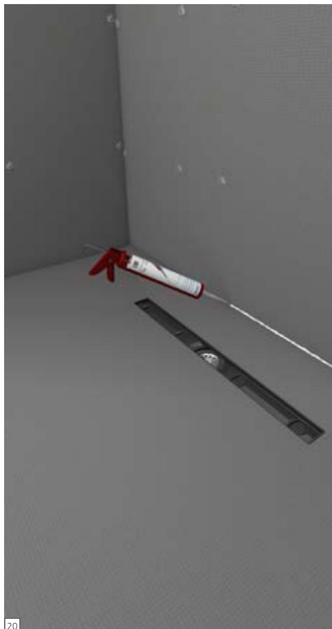
**EN** Apply continuous 1/2 in. beads of sealant between all connections of panels and install with tightly butted seams. Excess sealant must be spread flat with a putty knife. All seams and fastener heads in the assembly are covered with a topical 1/2 in. bead of sealant and spread flat. The seams should be covered 1 in. on either side of a seam. All fastener/washers are covered with sealant stretching 1 in. over the washer edges.
